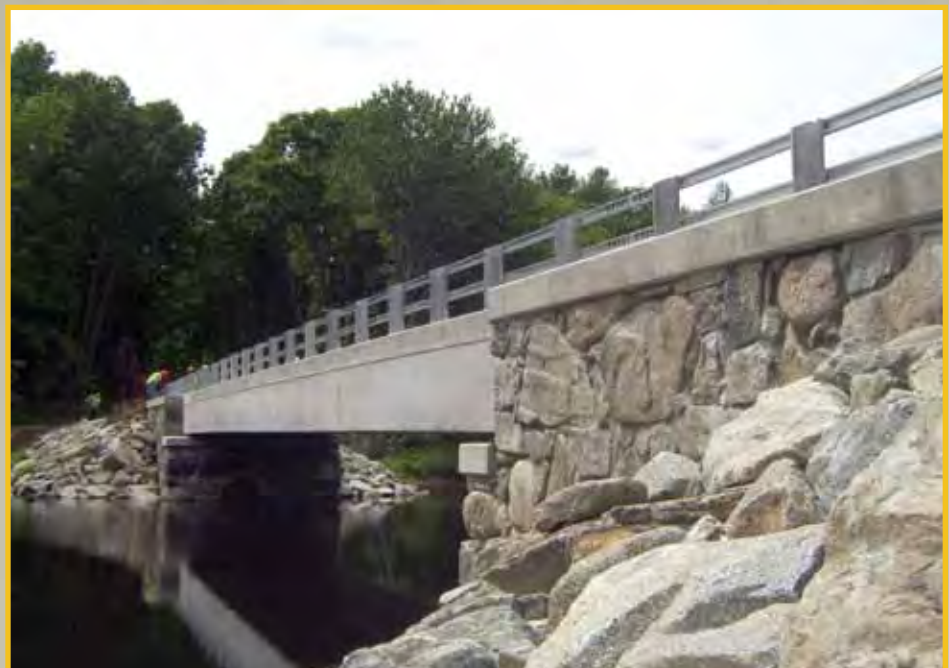
Wiswall Road Bridge Photo by David Costabile
