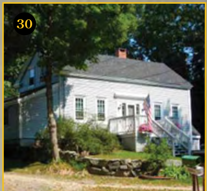
30 Wiswall Road All house photos by The Preservation Company
