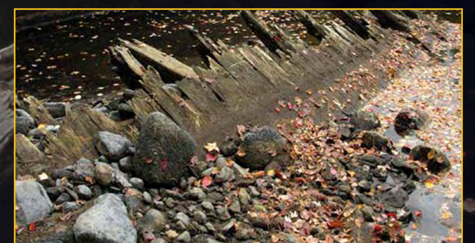
The remains of the previous wooden dam, usually covered by water, became visible here in 2009 when the level of the Lamprey River was lowered to allow for bridge construction.
