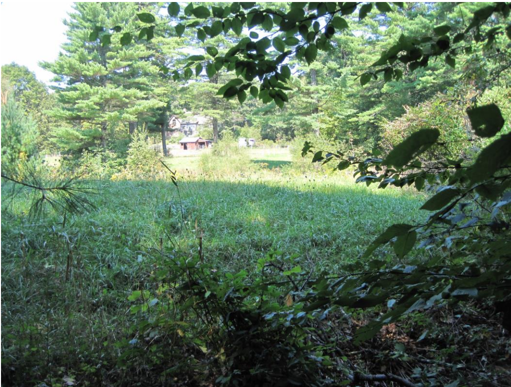
grassed earthen dam
