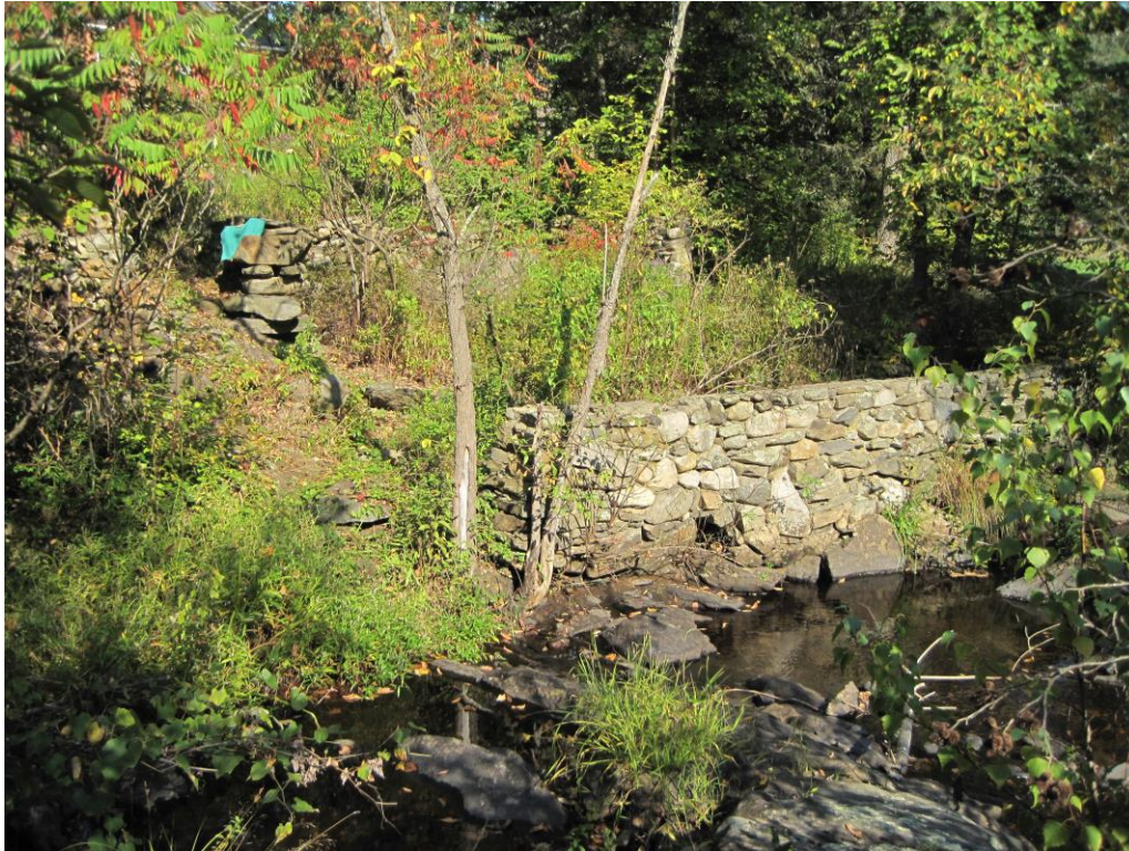
135.03 North River Dam
