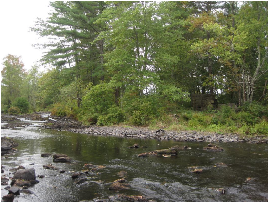
Remains of the mill structure can be seen on the right.
