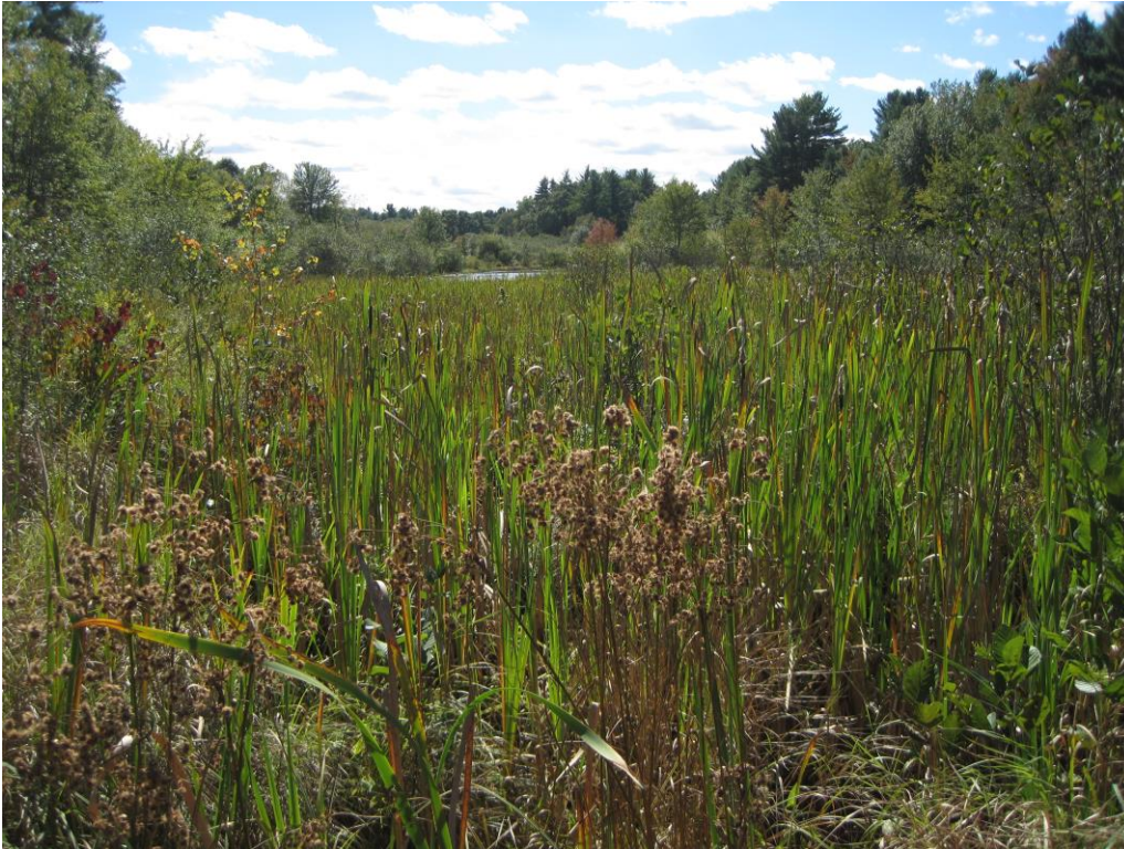
177.11 Dug Pond Dam – looking upstream from near former dam
