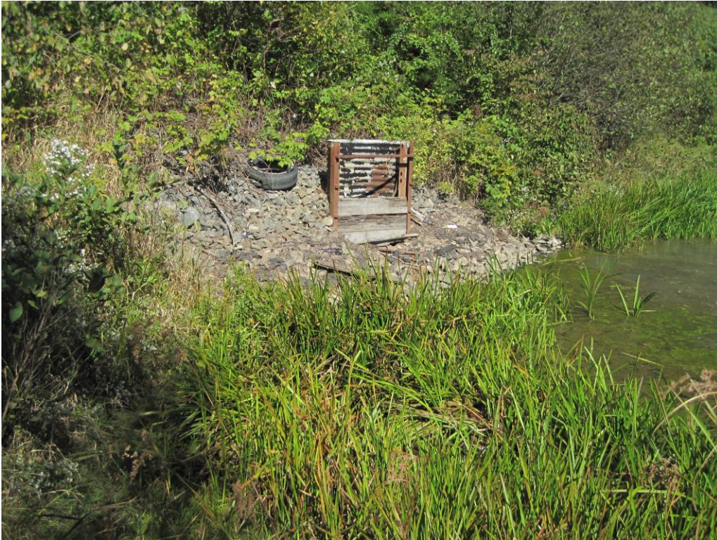
177.09 Wildlife Pond Dam spillway outlet
