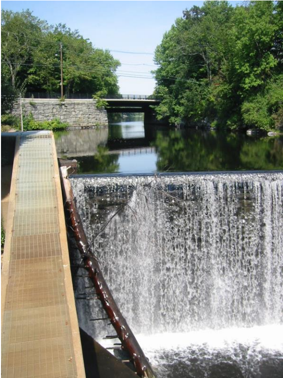
177.01 Macallen Dam with fish ladder on left, Rte. 108 bridge in background
