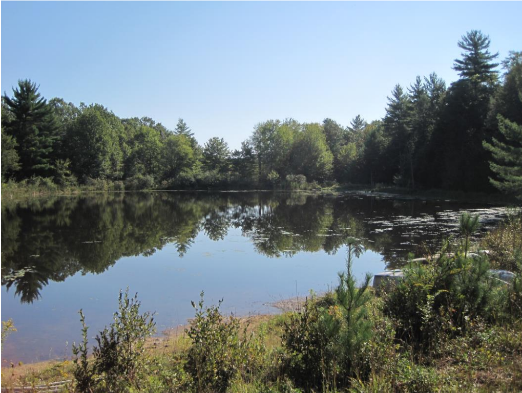
135.07 Recreation Pond – dam on opposite side of pond
