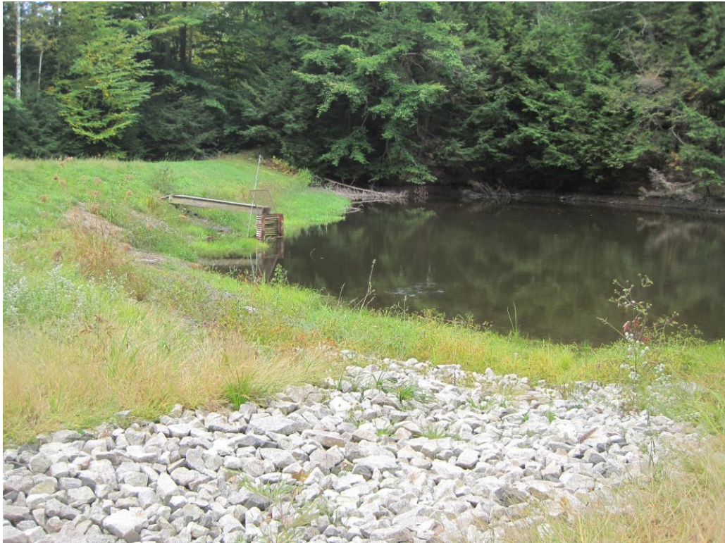
outlet to Conservation Pond
