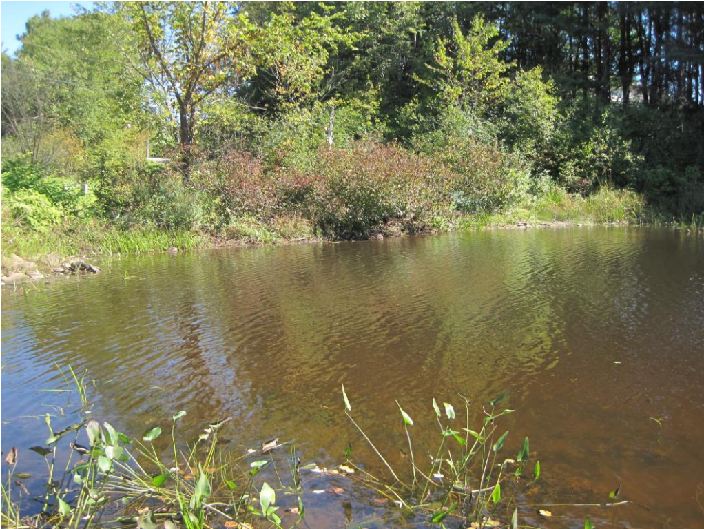
177.16 Recreation Pond Dam – looking to outlet at Grant Road
