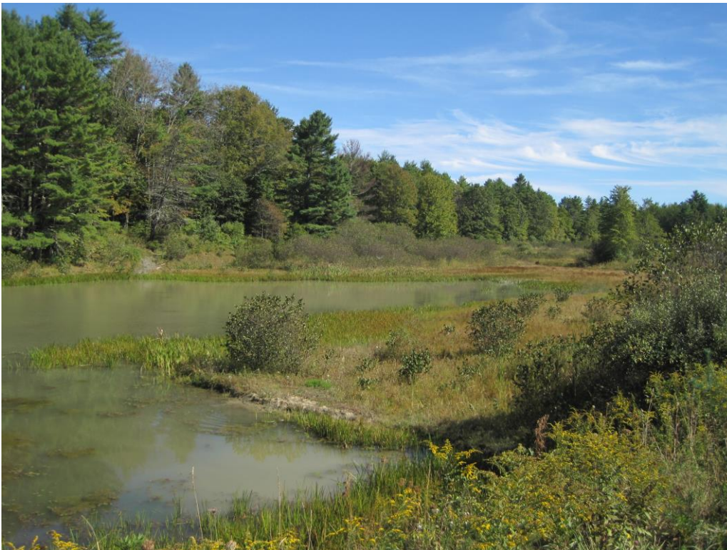
177.09 Wildlife Pond Dam looking upstream
