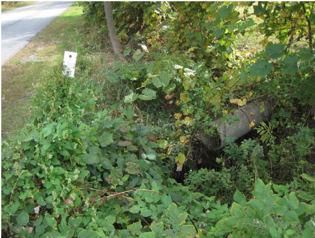
outlet to ditch next to Ash Swamp Road
