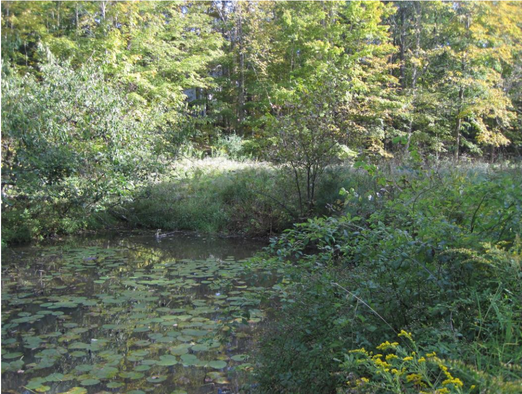
071.36 Stagecoach Farm Pond -view of dam from downstream, PVC pipe outlet
