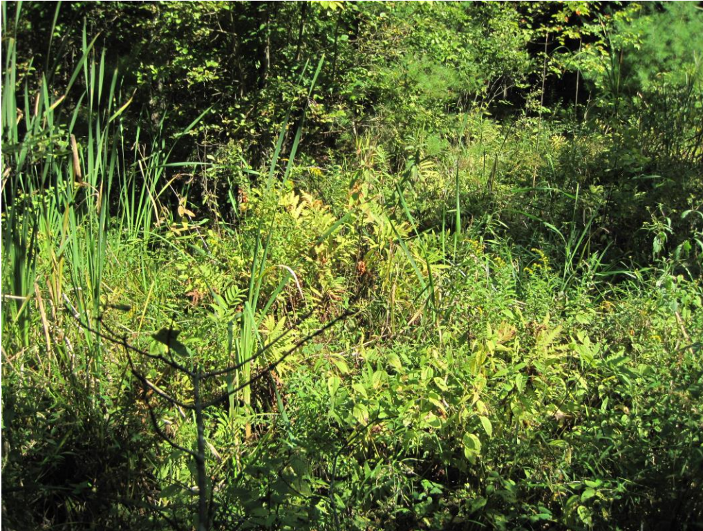
078.06 Bytne Dam – downstream of dam
