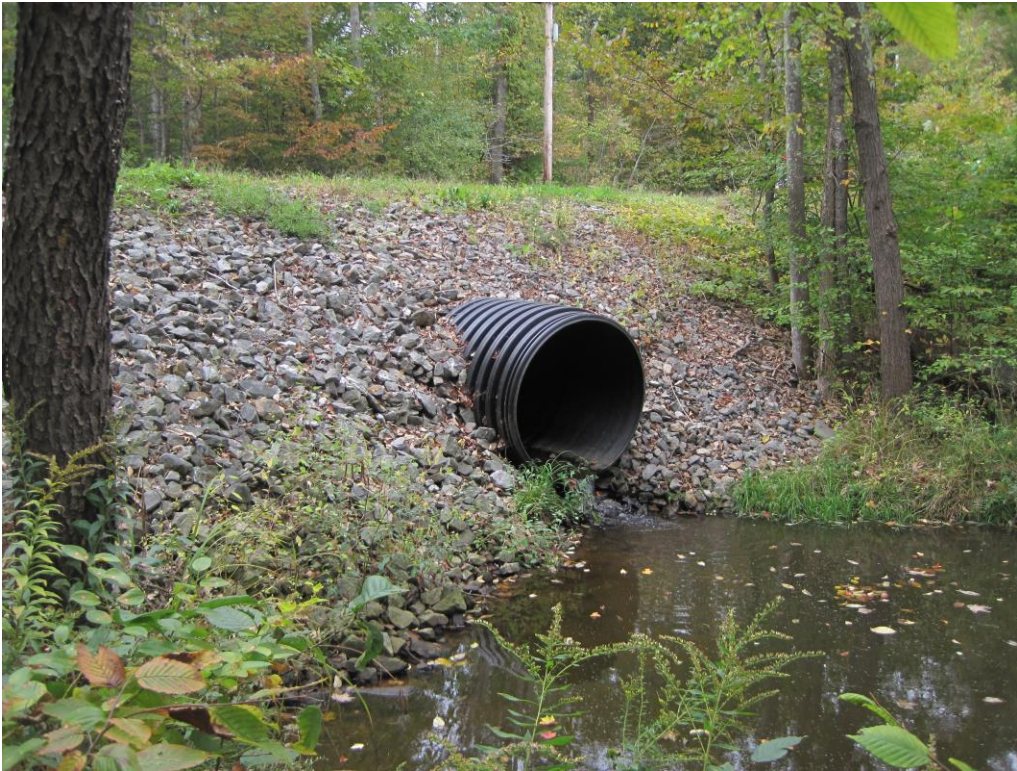
culvert on Lang Lane downstream from dam
