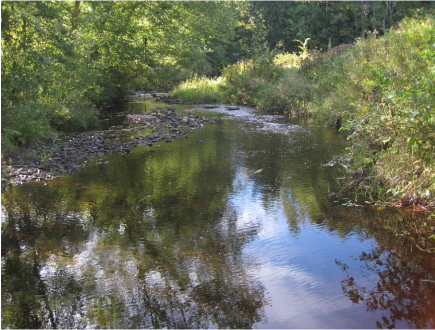
135.04 Thompson Little River Dam upstream view
