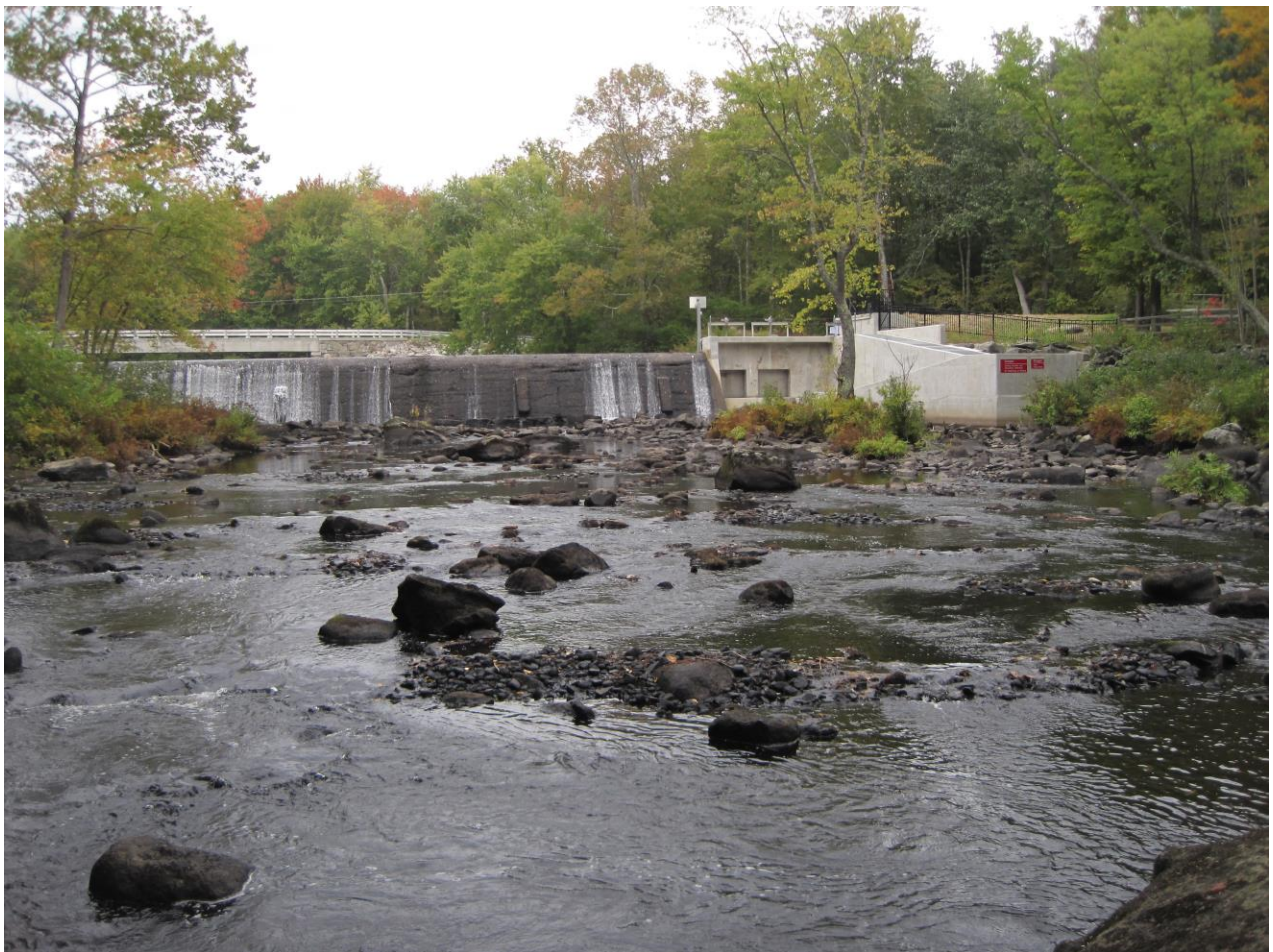
view of dam from downstream, fish ladder on right
