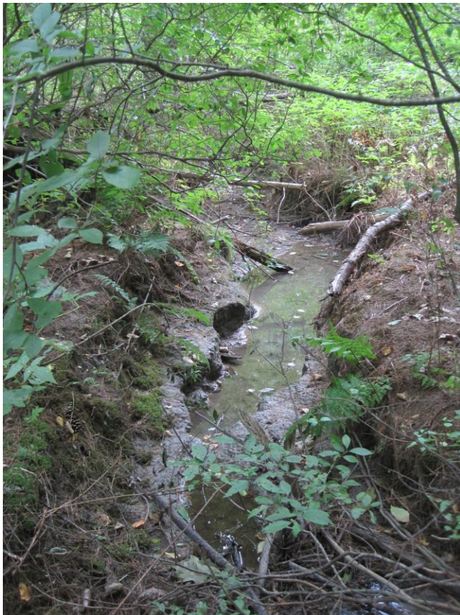
downstream of the dam
