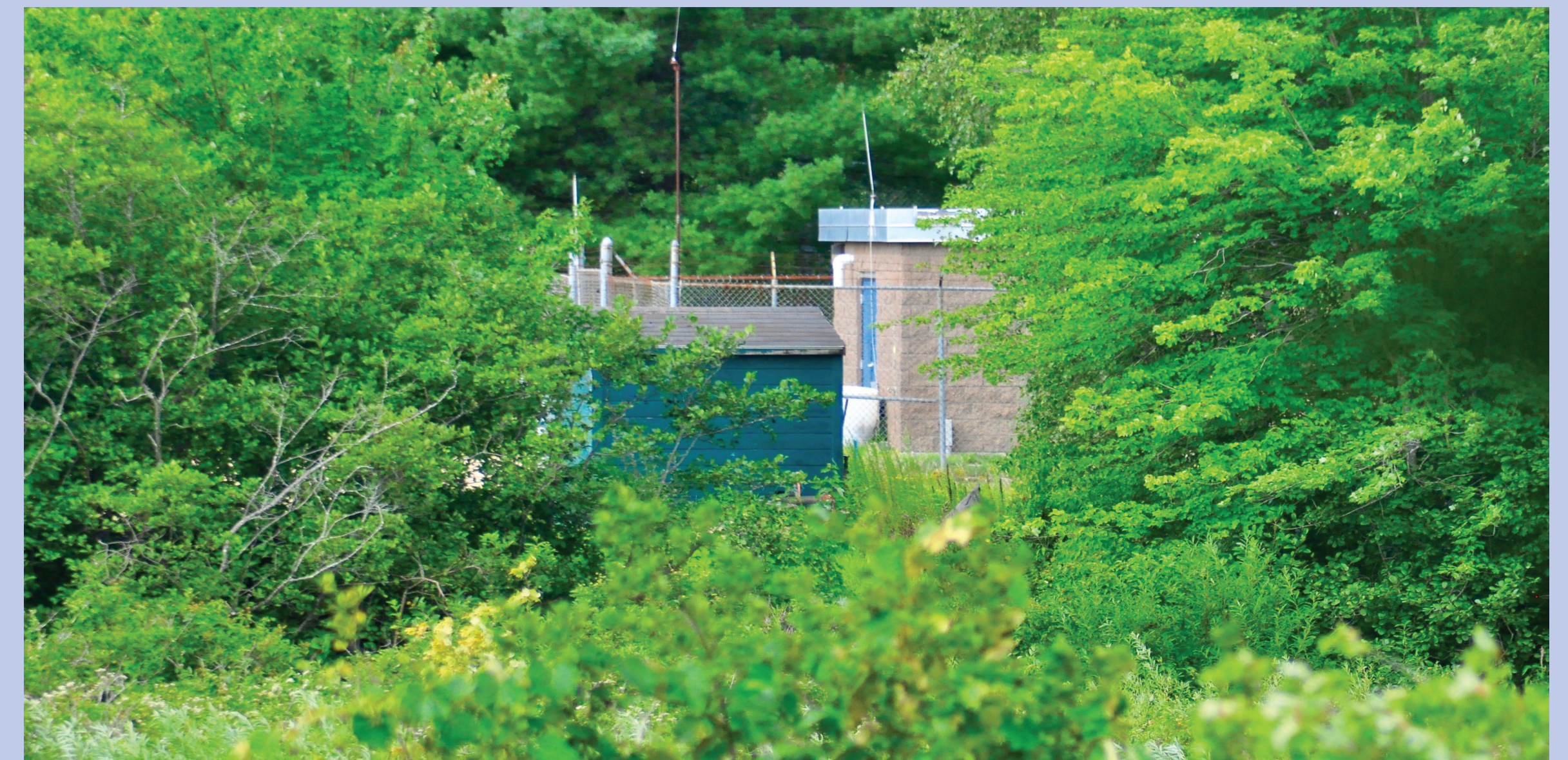
View of the drinking water treatment plant across the Lamprey River.
