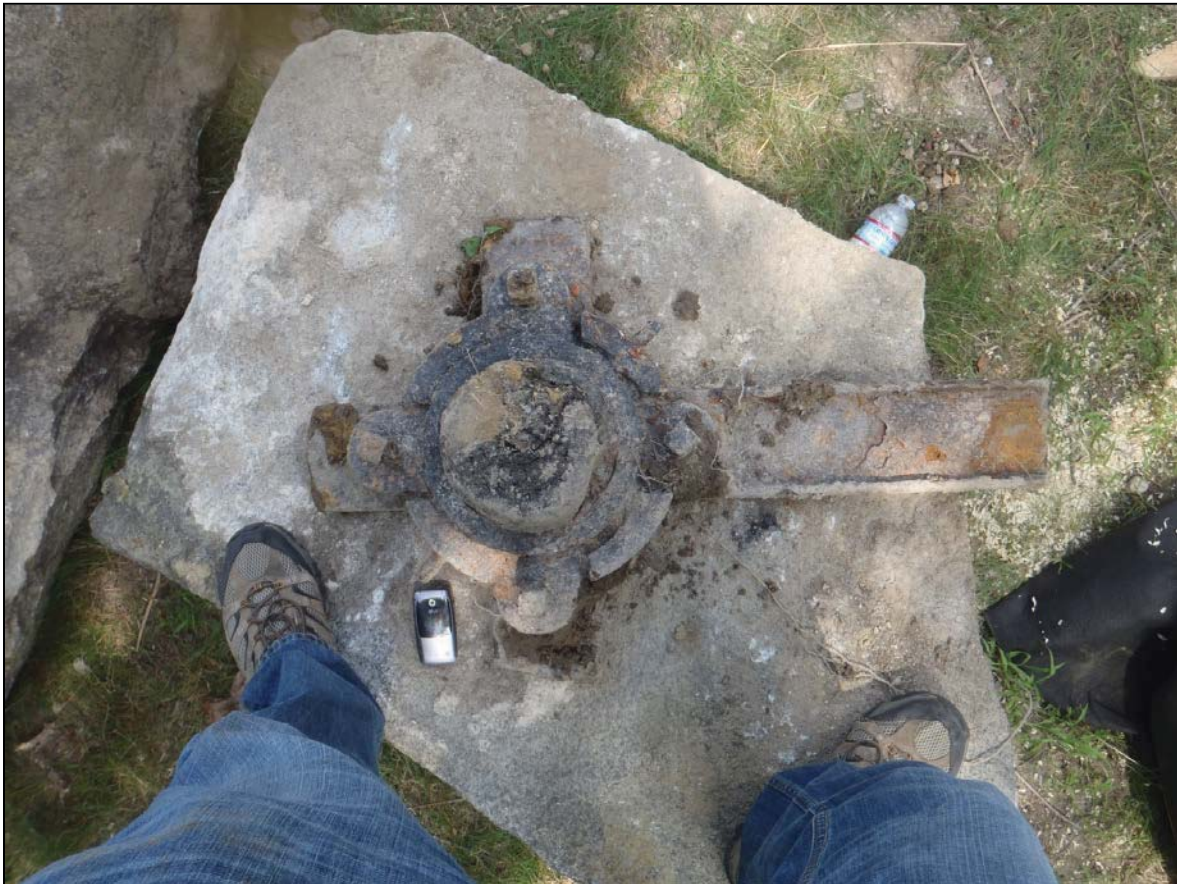
Top view of the drive shaft recovered from the Lamprey River during the 2011 fish passage construction project.
