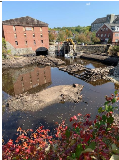
North wall Sept. 23, 2020. Note the old crib dam.
