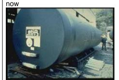
example of a double walled protected tank with leak monitoring equipment www.des.nh.gov
